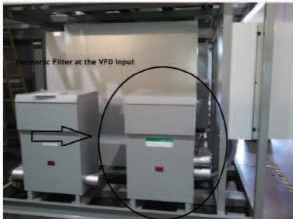
Harmonic Filter at the VFD Input and Sine Wave Filter at the VFD Output
